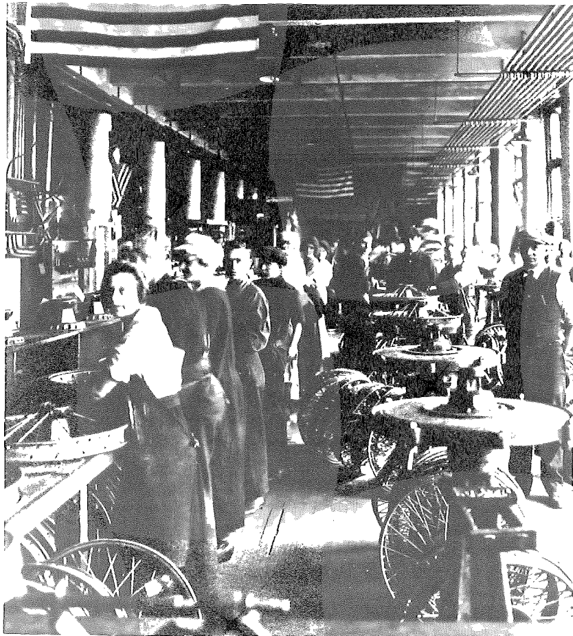
Fabricating steel-wire spoked wheels at Philadelphia plant in 1916. — Budd Photo.
