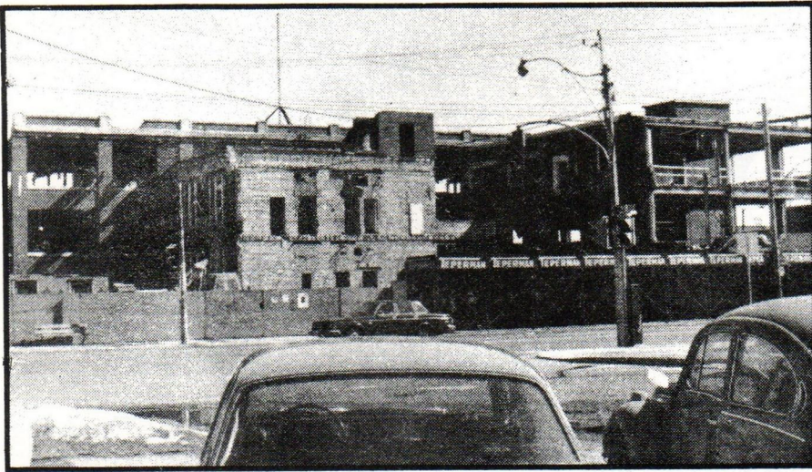
DEMOLITION of the Dominion Automobile plant on Laird Dr., this year.
